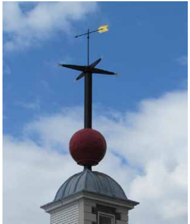
The Greenwich time ball on top of Flamsteed House Rory Walsh © RGS-IBG Discovering Britain
